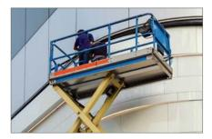
**Material handling:** Protect people working near shear points of scissor lifts, platforms and other equipment.
