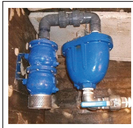
FloodSafe® Inflow Preventer with a Combination Air Valve
